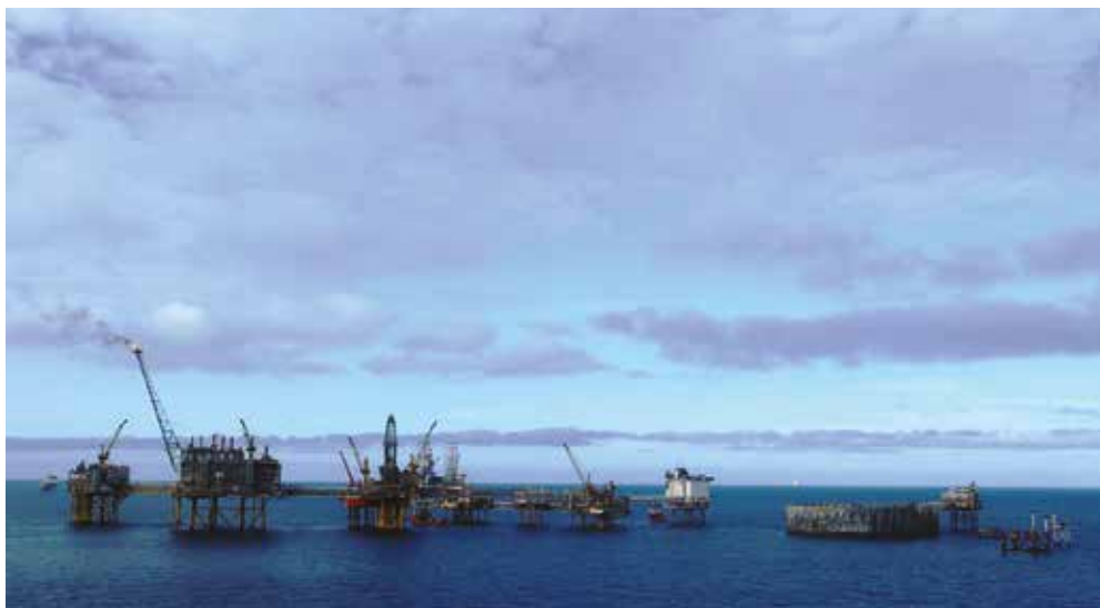
The whole offshore complex was threatened with a 6m subsidence
